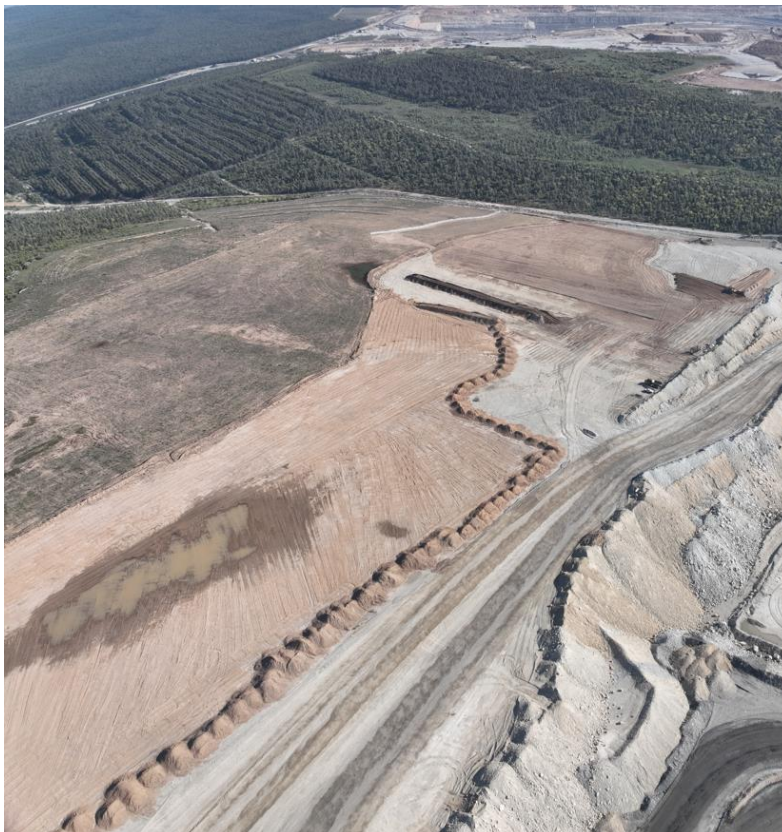
Figure 3 North Rehab – Subsoil being pushed out over recently landformed area (April 2025).
